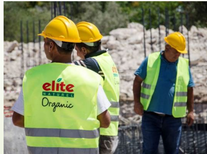
Building the foundation for a school in Eastern Turkey
